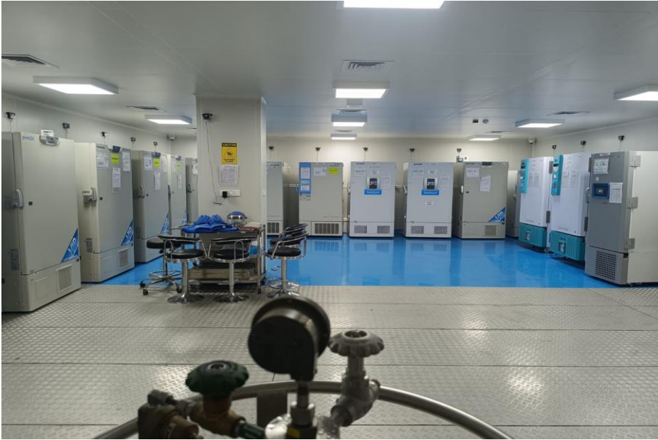
Figure 1: Ultralow deep freezers in the CBR
