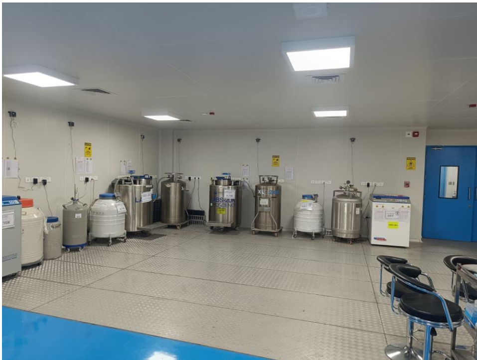
Figure 2: Liquid nitrogen storage systems in the CBR
